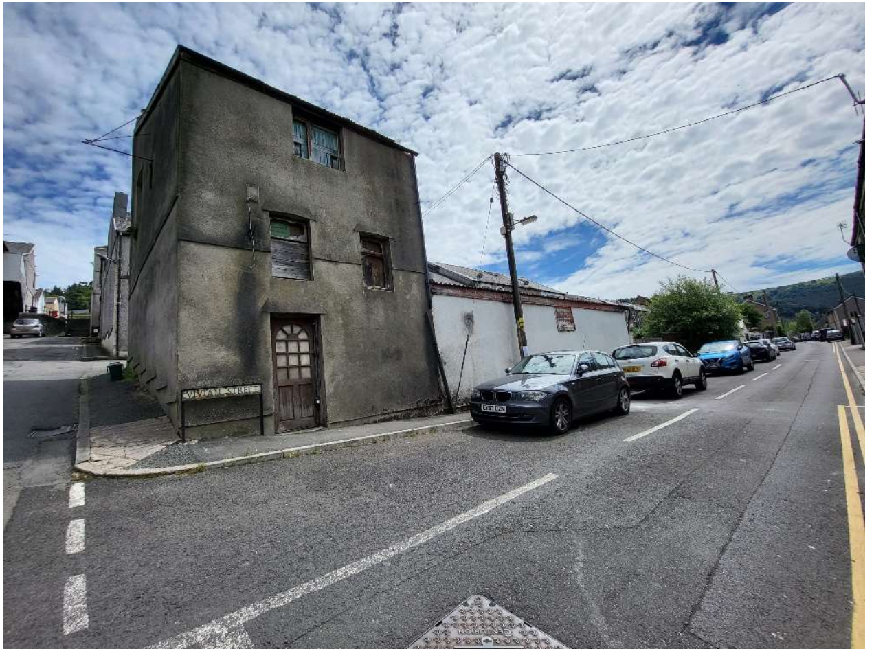
1.4 Figure 1.1 Existing Site from North Western Elevation (Vivian Street)
